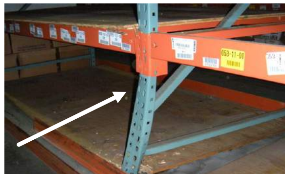
Damaged upright column
